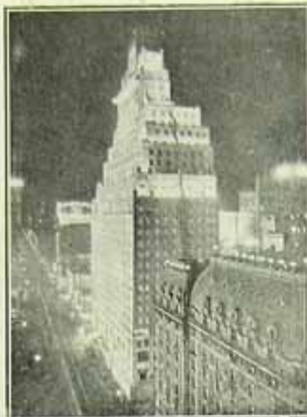
O Paramount Building
