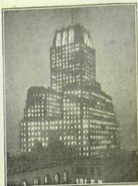
O Barclay-Vesey Building
