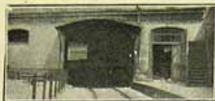
O tunnel da Central
